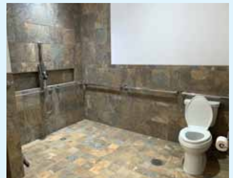
An open floor plan roll in shower which will accommodate a rolling shower commode chair, til-in-space shower commode chair, and shower attendant.
