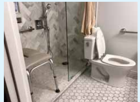
ADA height toilet turned to allow full side access for transfers including a grab bar for additional transfer assistance. This would be for an individual who is independent with transfers and does not need an over-toilet modification.
