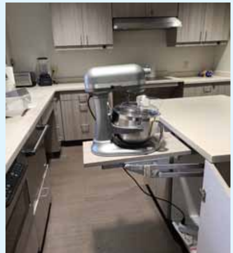
Roll Under Counter with Mixer Attached. The mixer is stored in the cabinet and more easily lifted into the use position with the adjusted rack.
