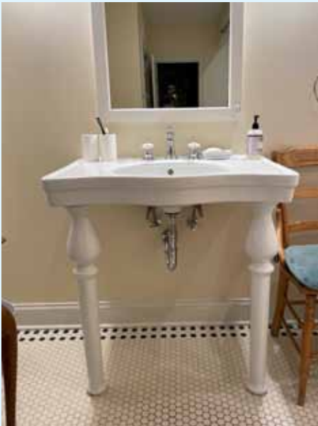
A pre-fabricated standard sink which is wide enough and high enough to allow for manual wheelchair roll-under access.
