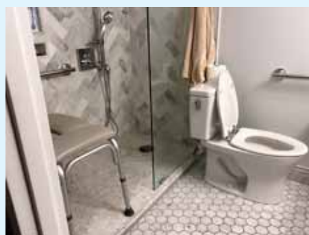
ADA height toilet turned to allow full side access for transfers including a grab bar for additional transfer assistance. This would be for an individual who is independent with transfers and does not need an over-toilet modification.
